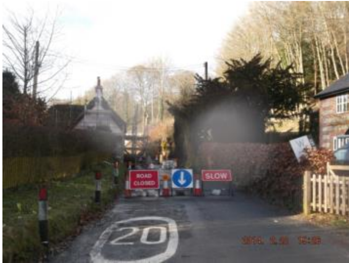
At Tollard Royal surface water flooding damage to a building required the road to be closed to traffic in 2014.
